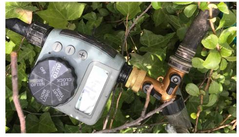
*Gazebo flowers* drip irrigation is controlled by a battery powered timer connected to the hose faucet in the middle of our oasis.
