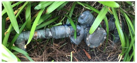
Valve handles aligned, horizontal: Valves open. (Barely visible).
